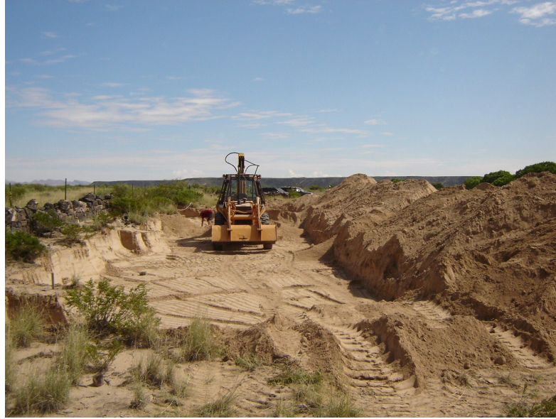
Figure 3.10. Backhoe removing overburden during 2007 excavations.
